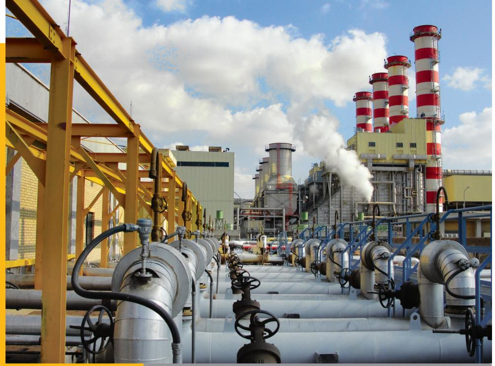
Qom combined cycle power plant with the capacity of 714 MW and area of 220 hectares is located in Qom province. This power plant has two combined cycle blocks including four gas units, made by Mitsubishi Company, with the nominal capacity of 128/5 MW each, and two steam units, made by ABB Company, with the nominal capacity of 100 MW each.
