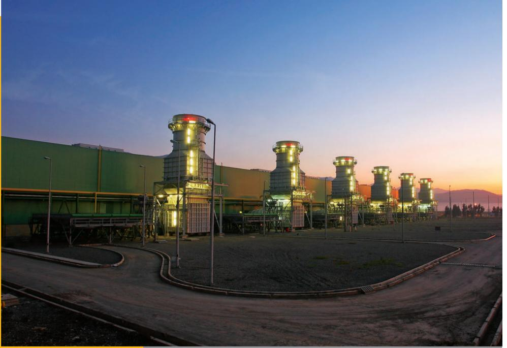
Ali Abad power plant with 1014 MW capacity is located in Ali Abad in Golestan province. This Power plant including six V94.2 gas units with 162 MW nominal capacity established in 2010.
